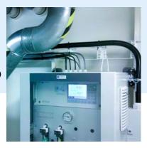
The complete system for continuous maritime emission measurement as per MARPOL regulations
